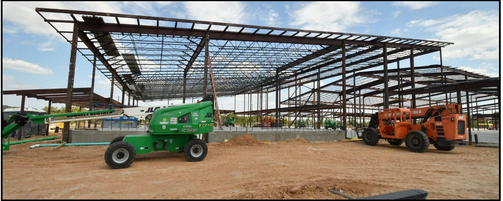
Joists and Metal Decking in Progress at Gym/Cafeteria
