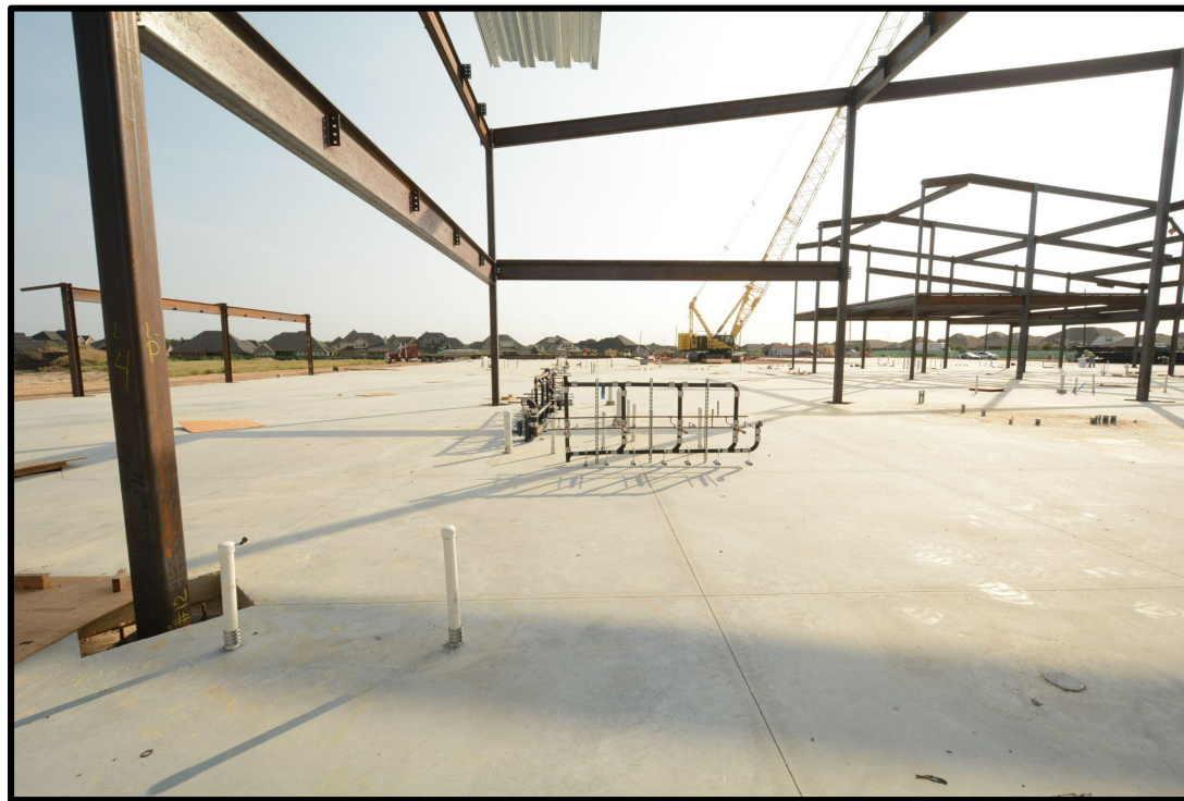
Plumbing Carriers Installed
