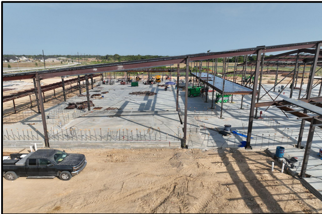
Steel Erection with Deck Installed
